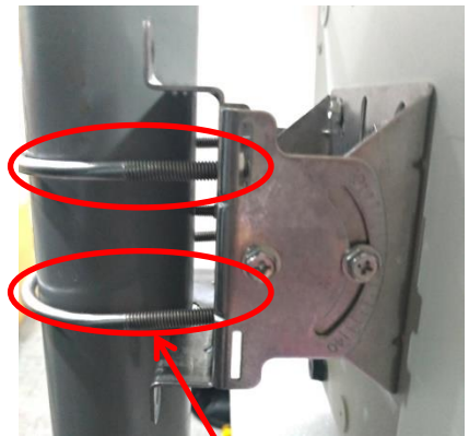
Fasten Tightly to the Pole When the U-screw is Fixed, Please Lock Parallel Width Fixed
